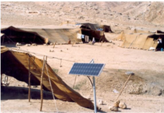
Figure 9: PV lighting Bedouin system
