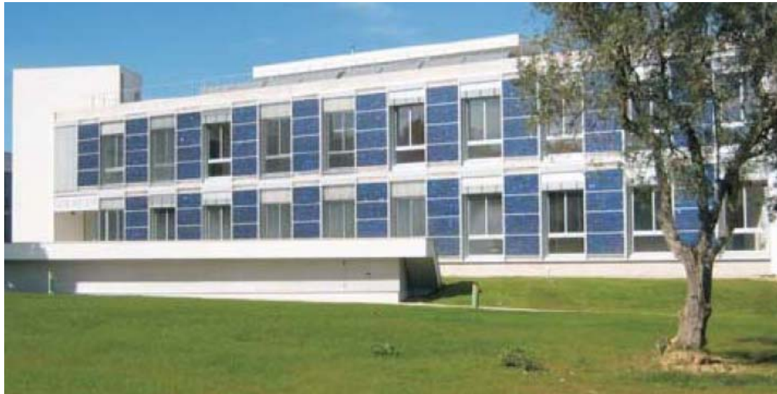
Figure 45. Integration of photovoltaics on the southern façade of Solar XXI Building in the INETI Campus in Lisbon [source: ADENE]
