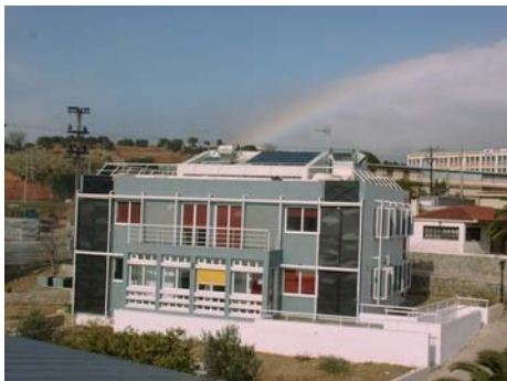
Integration of PV and thermal solar systems on the building envelope of the bioclimatic building of CRES in Pikermi, Greece
