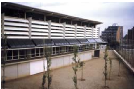
Use of thermal solar systems as external shading devices on the façade of the Poliesportiu Municipal del Guinardó Torrent d'En Melis, Barcelona, Spain
