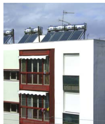
Figure 52. Examples of solar heating installations in Greece [source: CRES]
