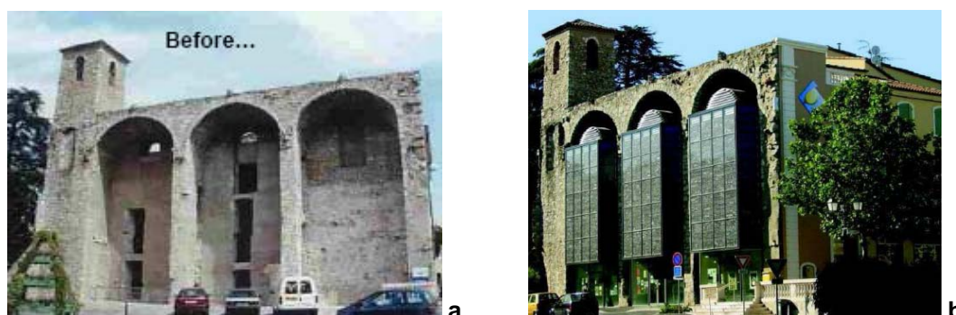
Figure 40. The 11 th century monument in Alès, South France, whose arcades have been covered with 10kWp PV panels [source: ADEME]
