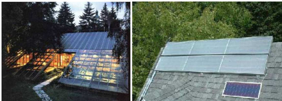
Figure 46. Examples of solar heating and photovoltaic installations in individual houses in Portugal [source: ADENE]
