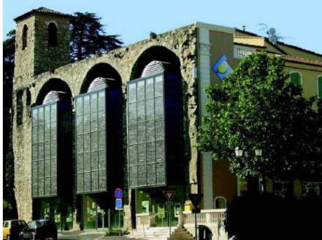
Integration of PV panels on the façade of an 11 th century monument in Alès, South France
